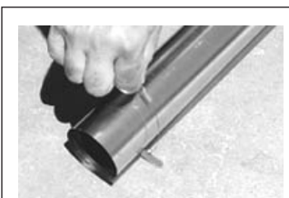
Slide on the retainer ring about one inch above cinder screen slots
